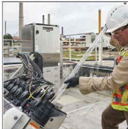
Figure 4. Operator changes UV bulb.
