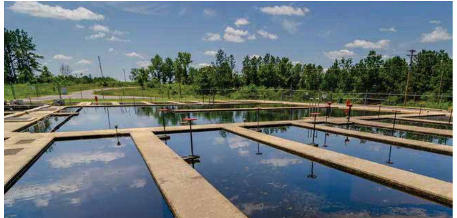
Settling basin at Russellville, Alabama, water treatment plant.
