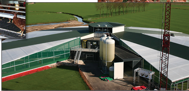
Like spokes of a wheel, the quadrants of the Rondeel egg production system radiate out from a central core used for delivery of feed and packing material and transfer of farm-packed eggs.
