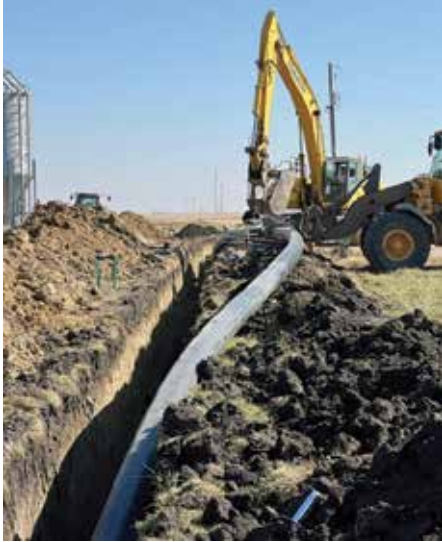
HDPE pipe is flexible enough to be installed in trenches, by plowing or by any trenchless method. Photo courtesy of ISCO.
