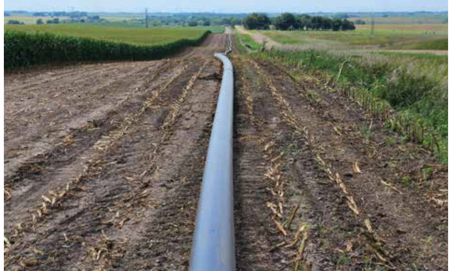
Heat-fusing 53-foot-long lengths of HDPE pipe constructs a monolithic, leak-free pipeline. Photo courtesy of Douglas Westerman/ORWS.
