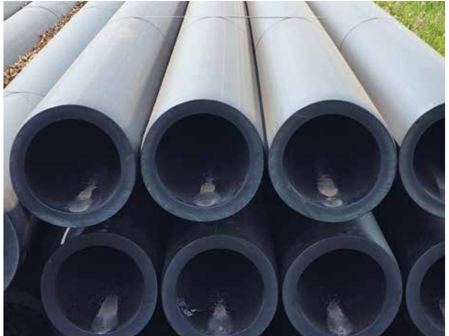
Load of 12-inch HDPE pipe ready for fusing and installation. Photo courtesy of Douglas Westerman.
